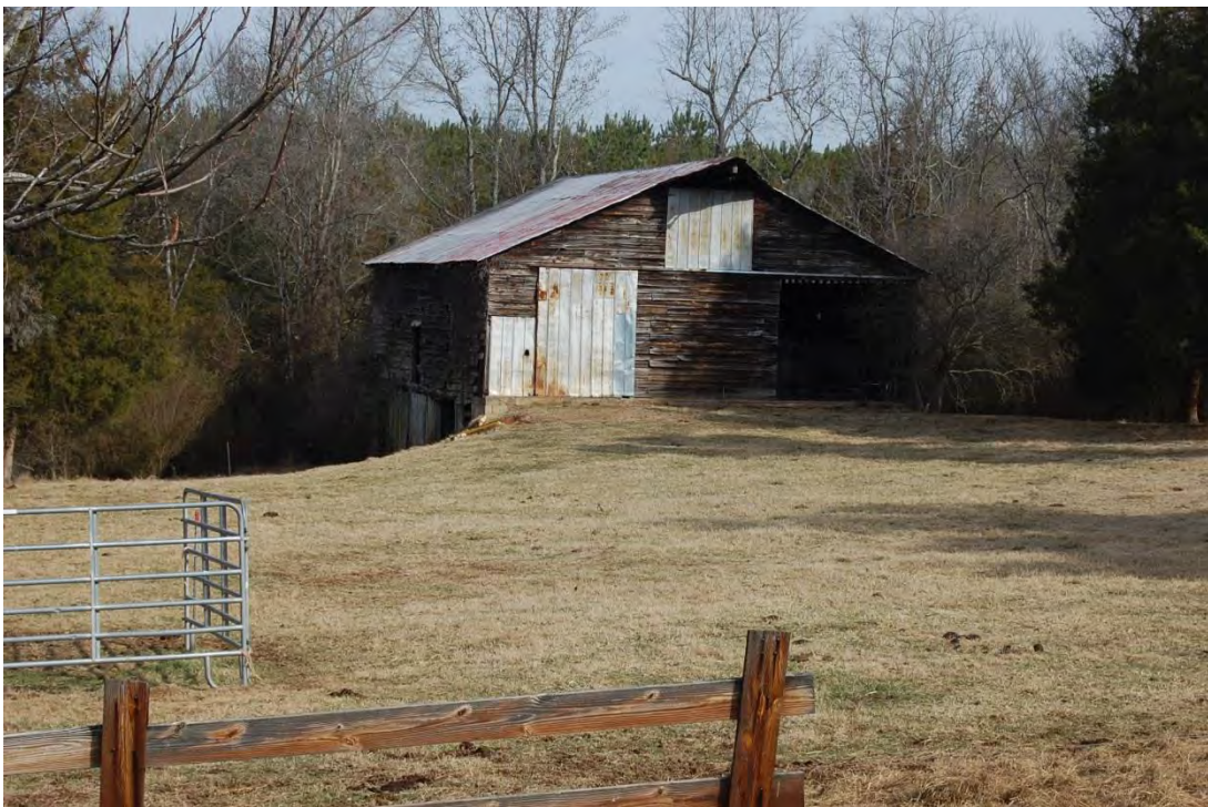
John Mathias Barnhardt House, Barn, Looking North.
