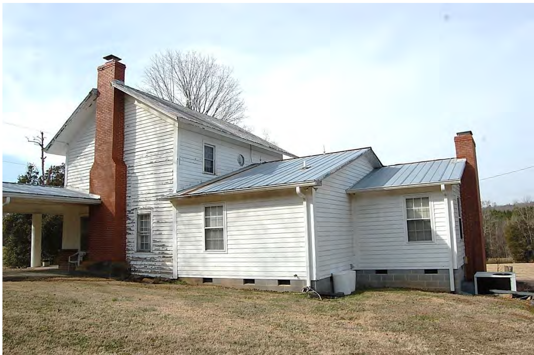
John Mathias Barnhardt House, Side (East) Elevation and Rear Ell, Looking West.
