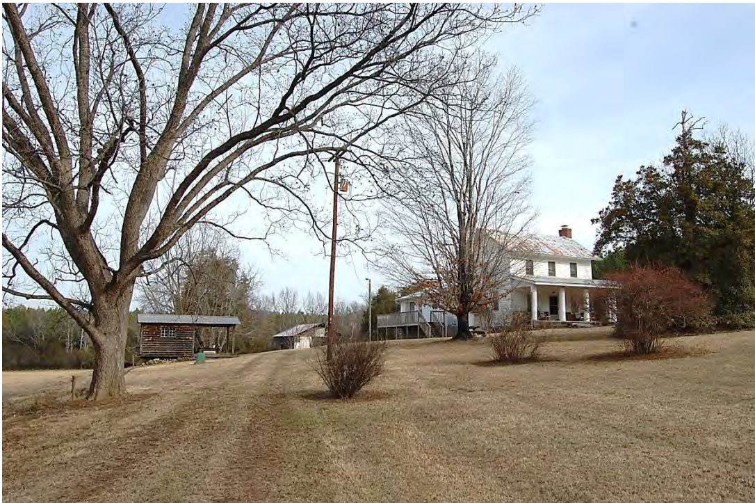
John Mathias Barnhardt House, Overall View of House, Barn (Background), and Well House (Left), Looking Northeast from Little Bear Creek Road.
