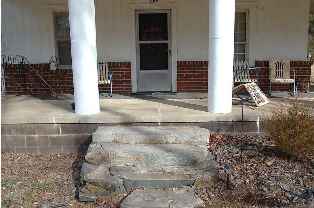
John Mathias Barnhardt House, Detail of Front Porch With Original Slate Steps.
